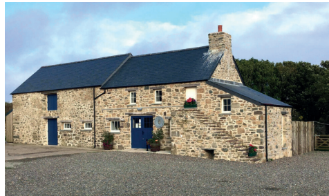
The Old Farmhouse Brewery after refurbishment
